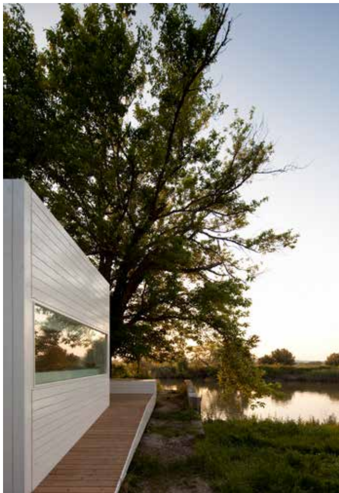
treehouse | engineered by JULAR
