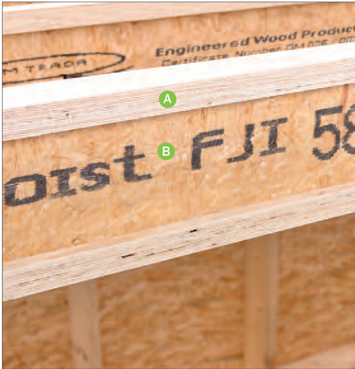
A Flange manufactured from Kerto®. B Web manufactured from high quality OSB.
